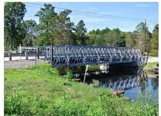
The deficient structure was replaced with a 70-foot-long by 24-foot-wide Acrow panel bridge with a TL-2 guide rail. Both Acrow bridges include deck panels that distribute loads efficiently, with an epoxy aggregate non-skid deck surface that is durable and long lasting.
