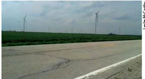
*The flexible pavement on this county road near Gifford, IL, shows signs of distress (visible cracking). The road services the adjacent wind farms visible in the distance.*
