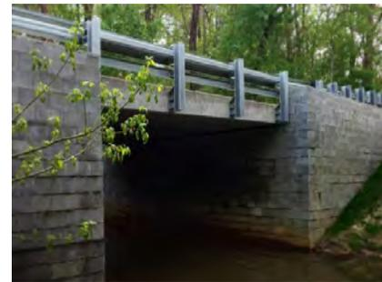
*New Jersey's first GRS-IBS project replaced a flood-damaged bridge in Gloucester County.*
