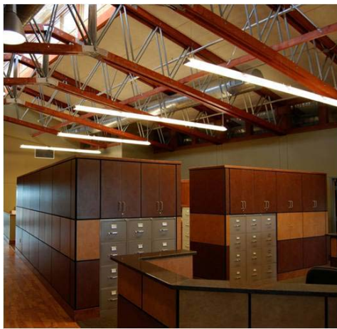
T-5 Florescent Light Fixtures
